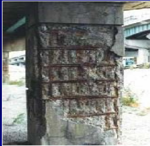
(ASR) Environmental Damage (Corrosion)
