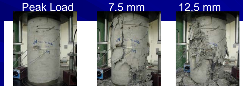
Concrete: extensive spalling
