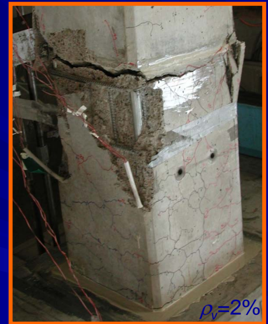
Reinforced Concrete Hinge Region After ~2% drift
