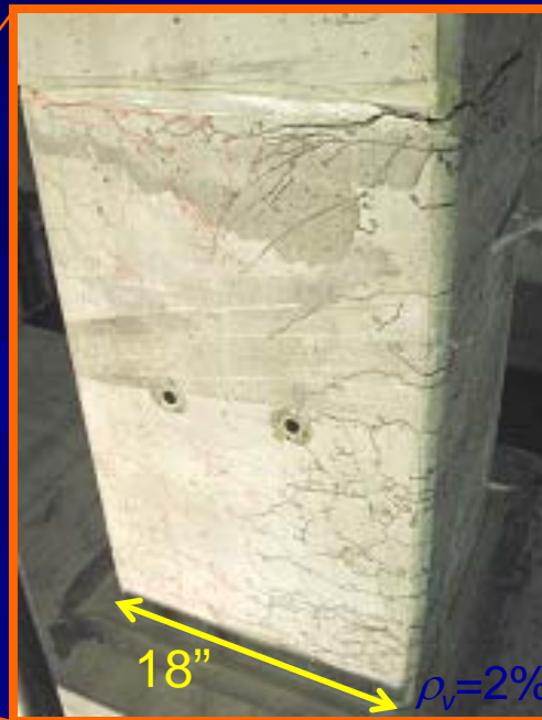
ECC Hinge Region After ~4% drift
