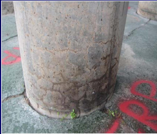
(ASR) Environmental Damage (Corrosion)
