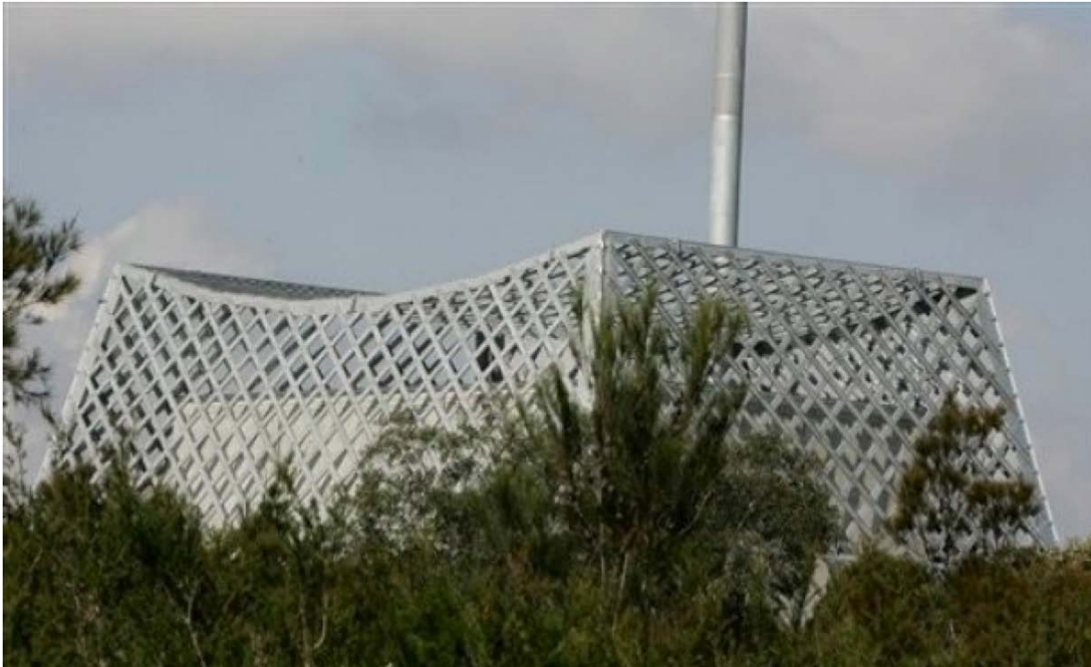
Lucas Heights reactor, Australia, with a steel-girder external event shield
