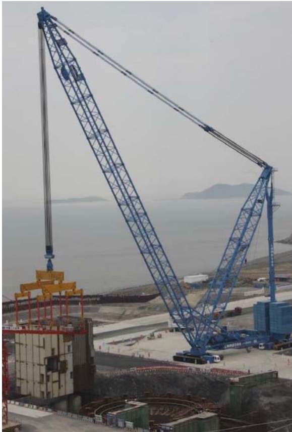
770-ton AP-1000 auxiliary building module, assembled from factory prefabricated plate components, being set in place onto foundation, Sanmen, China, July 2009
