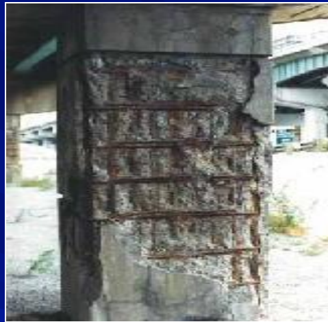
(ASR) Environmental Damage (Corrosion)
