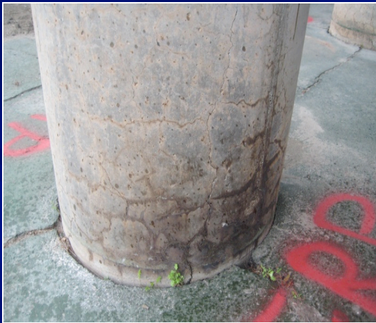
(ASR) Environmental Damage (Corrosion)
