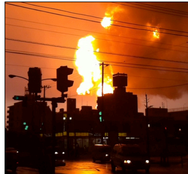
Fire at the Cosmo Oil refinery in Ichihara, March, 2011
