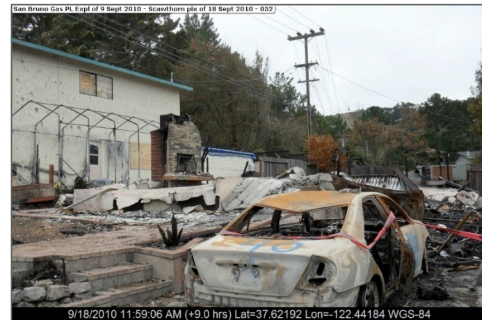
Damage scene (Prof. Charles Scawthorn)
