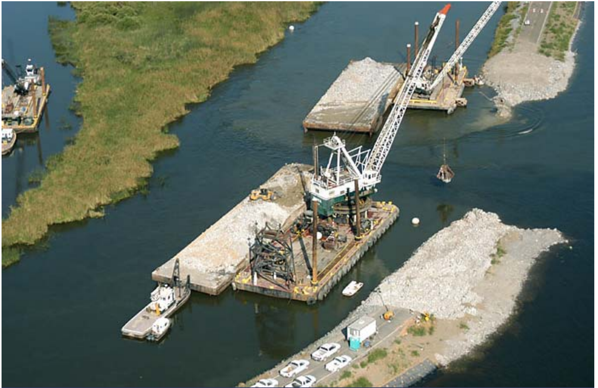
Closing Levee Breach
