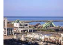
Haramachi thermal power plant (Minami-soma, Fukushima)
