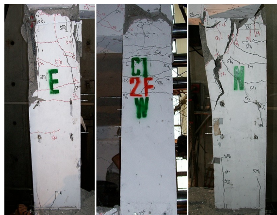
Fig. 23. -3% 1 st cycle: C1-2F shear failure
