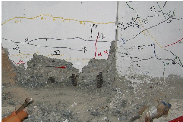
Fig. 20. -2% 3 rd cycle: C6-1F rebar buckle.
