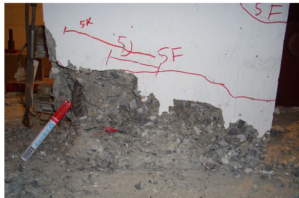
Fig. 21. +3% 1 st cycle: C1-1F rebar buckle
