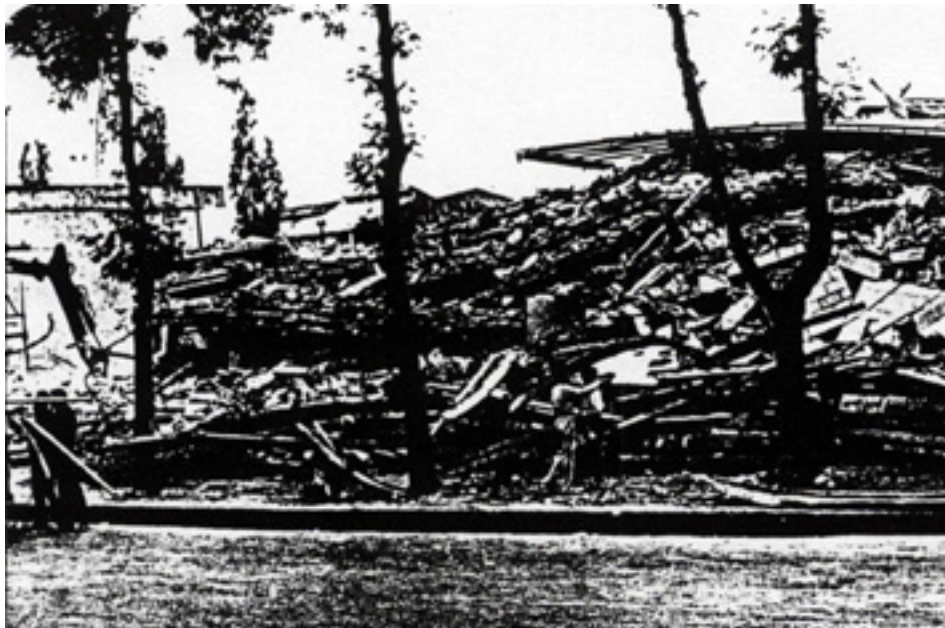
Fig. 2. A typical failure of Khorjini connection in Manjil Earthquake
