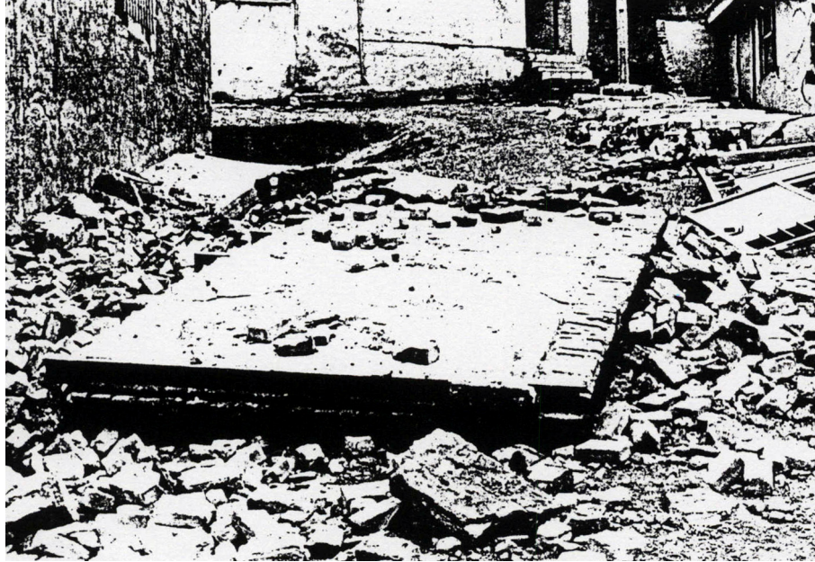
Fig. 3. A typical roof failure in Manjil earthquake
