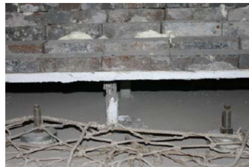
Fig. 14 Concrete flaking off on the bottom floor column
