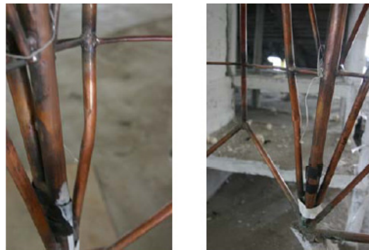
Fig. 12 Pits on the support members
