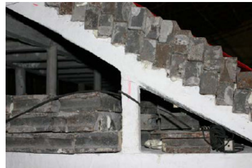
Fig. 8 Cracks on the 4 th floor column
