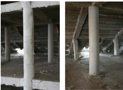
Fig. 13 Cracks on the 4 th floor column
