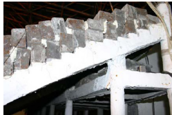
Fig. 10 Cracks on the boundary beam
